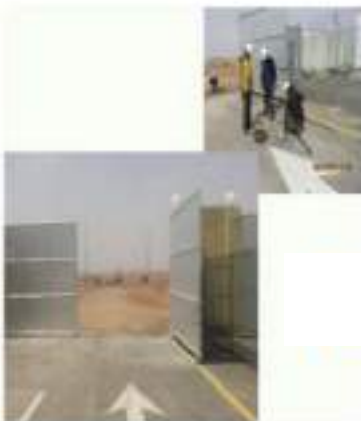
Installation Of Rail For Main Gate Works
