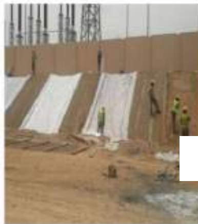
Slope Protection Works
