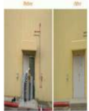
Door Paint at Substaions
