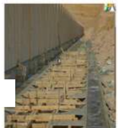
Drain Channel Works
