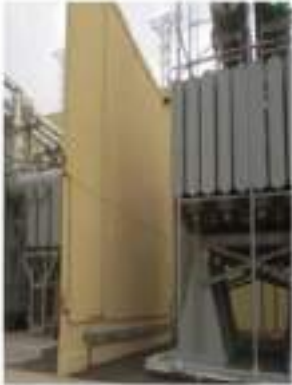
Fire Wall Painting Works
