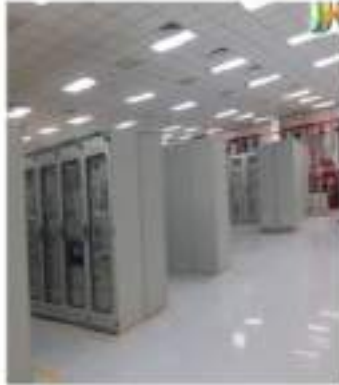
False Ceiling Works
