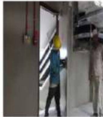
Doors Final Alignment And Installation
